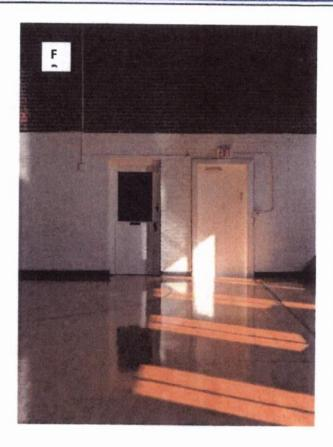
These four doors (two on each side of the gym wall here) will be replaced with new metal doors with current safety hardware and glass lights to pass vision dimension standards. Outside door of the two, on each side, will be enlarged to approximately 40".
