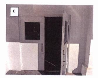
Two entrance door systems that currently exist at the west entrance are dated and require said updates and safety mechanisms to insure proper access and egress with panic hardware, proper vision light (glass) dimension with safety elements and thresholds to withstand traffic and be weather resistant.
